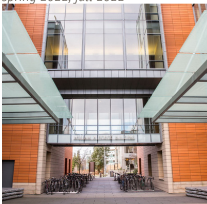
12. Foegen Building Skybridge spring 2022, fall 2022
